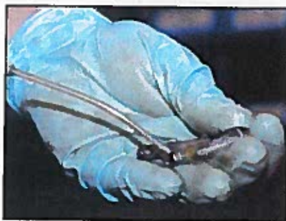
It is important to lubricate the threads as well as the head of all fasteners before torquing down.
